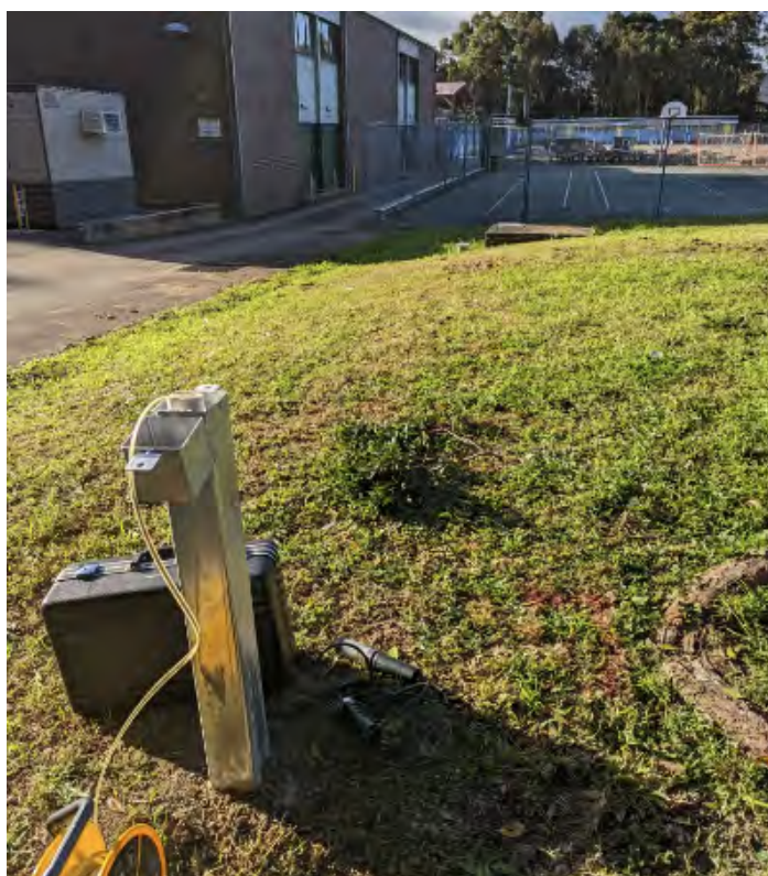
Photo 6: 28/06/2022 - MW01 location on the mound south of the site, looking north.
