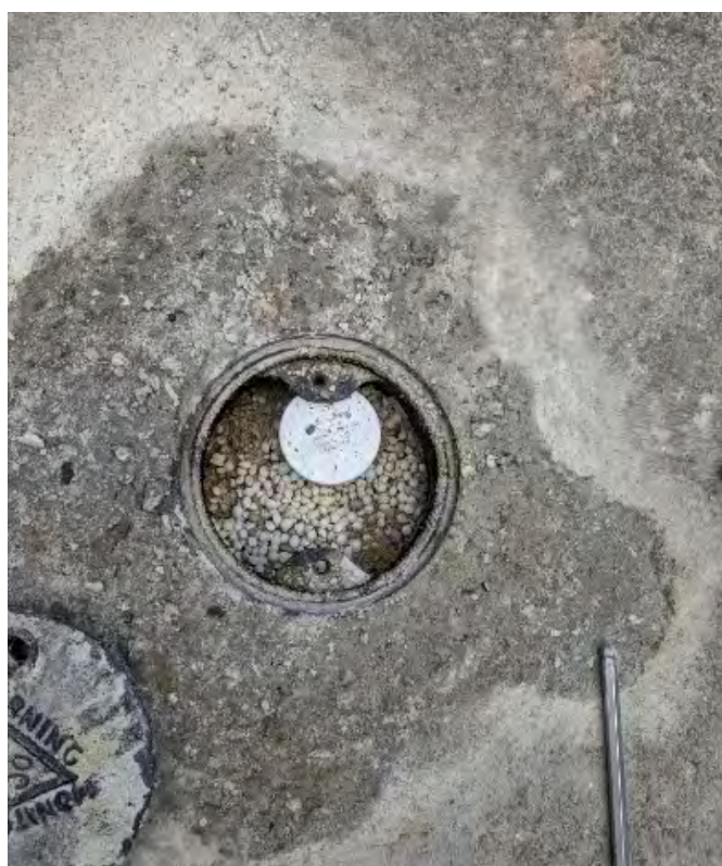
Photo 8: 28/06/2022 - MW03 location in the car park in the south of the site.
